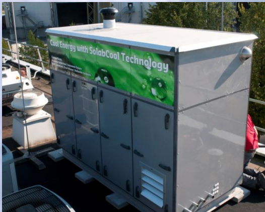
Cooling office building AVR driven by waste heat from own incineration plant.
